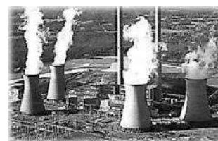
Evaporation cools hot water produced by power plants
